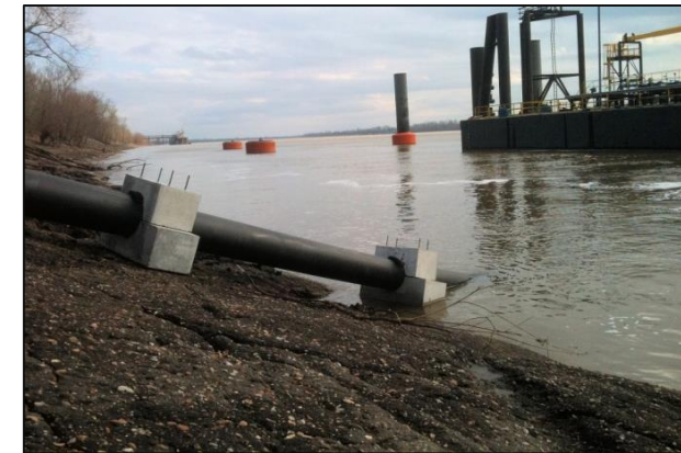
Outfall Line: HDPE Piping
